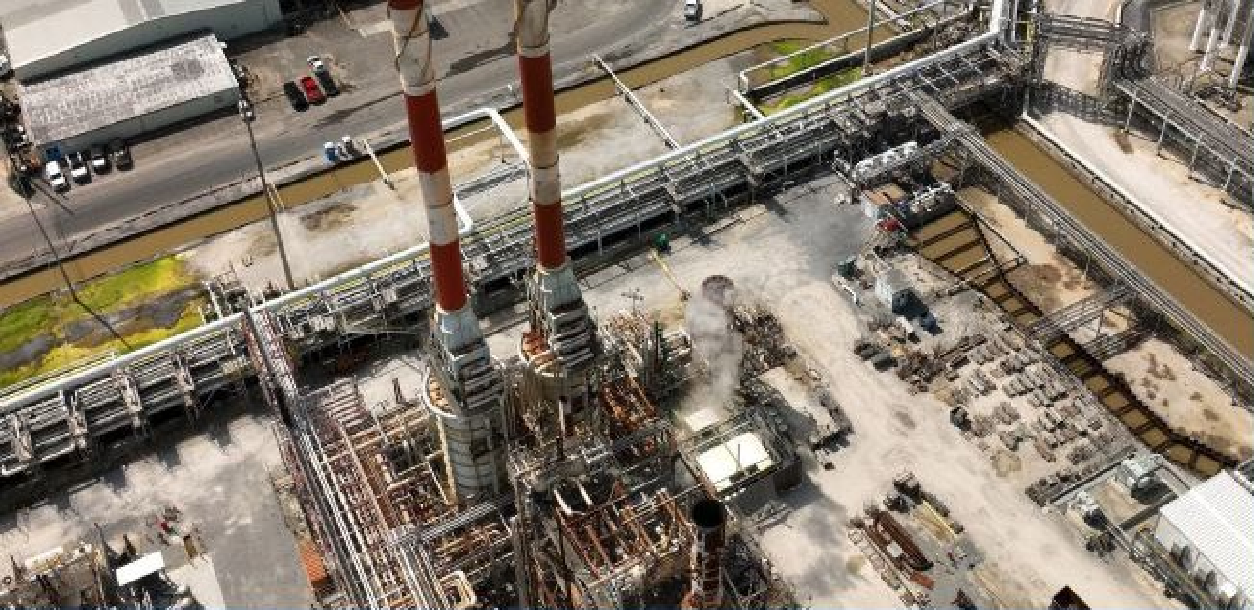
Image 51: still from recovered DJI Mavic 3 video dated 21 February 2023 showing the Dow Chemical plant in Hahnville, LA. Video taken during FLY0120 .
