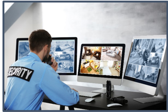
Figure 6: Security team monitors CCTV Source: Shutterstock
