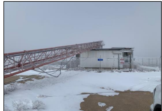
Figure 9: 643-foot tower in Notrees, Texas, damaged by winter storm Uri.
